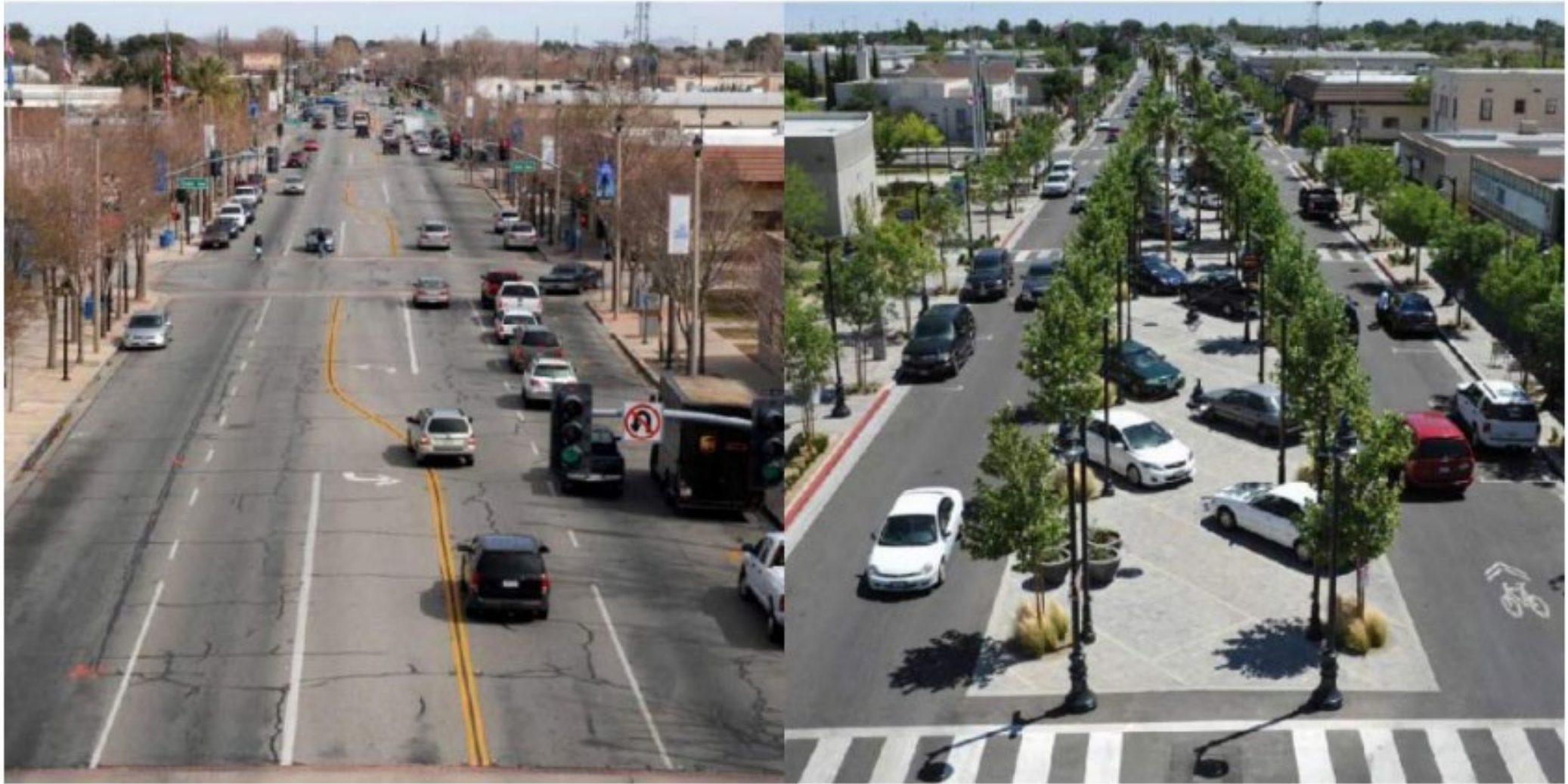
Above: Lancaster Boulevard (Lancaster, CA) before road diet (Left) and after road diet (Right). Image accessed from Project for Public Spaces. Below: Preferred Bikeway Types Graphic. Image accessed from Ohio Department of Transportation.
